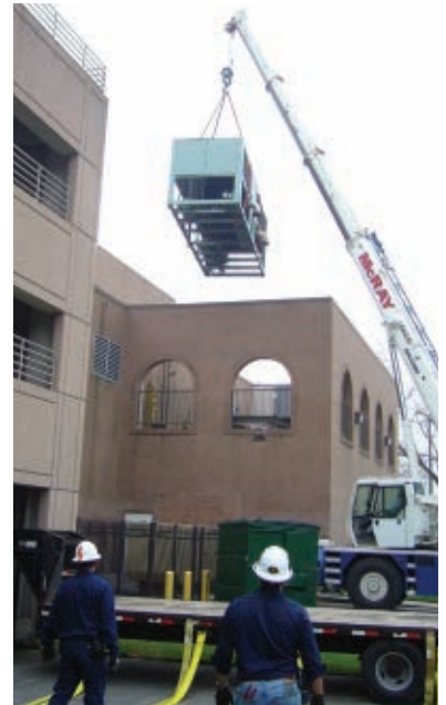
Seven of the buildings received HVAC upgrades. Old rooftop units and split systems were replaced by new, high-efficiency units.
